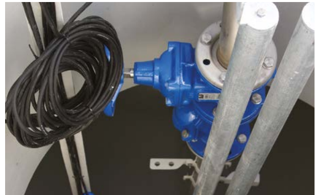
The pump can be raised up in the pump shaft.
